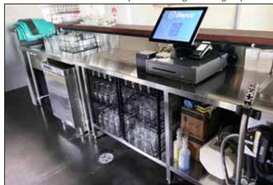
610mm deep bench with 610mm sink and dishwasher underneath.
